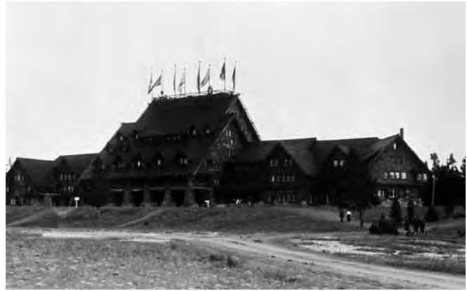
The roof shingles of the Old Faithful Inn, shown here in 1912, were originally coated with a red mineral paint believed to hinder flammability.
