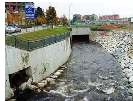
Tunnelling of Seveso River
