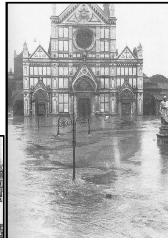
Flood in Florence in November 1966
