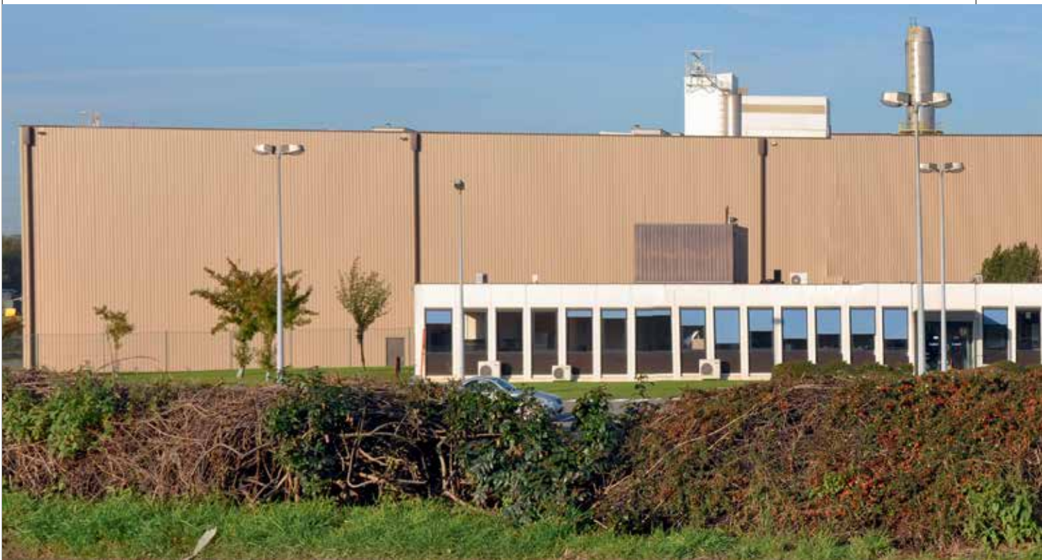
▲ The Visé plant in Liège province
