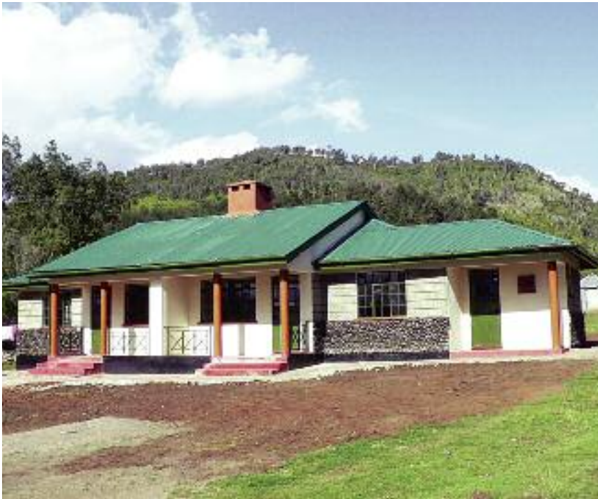
The recently completed guard post in Nandarasi. Aggreko donated Kshs 4 million to the construction of this guard post as part of the fence maintenance process.
