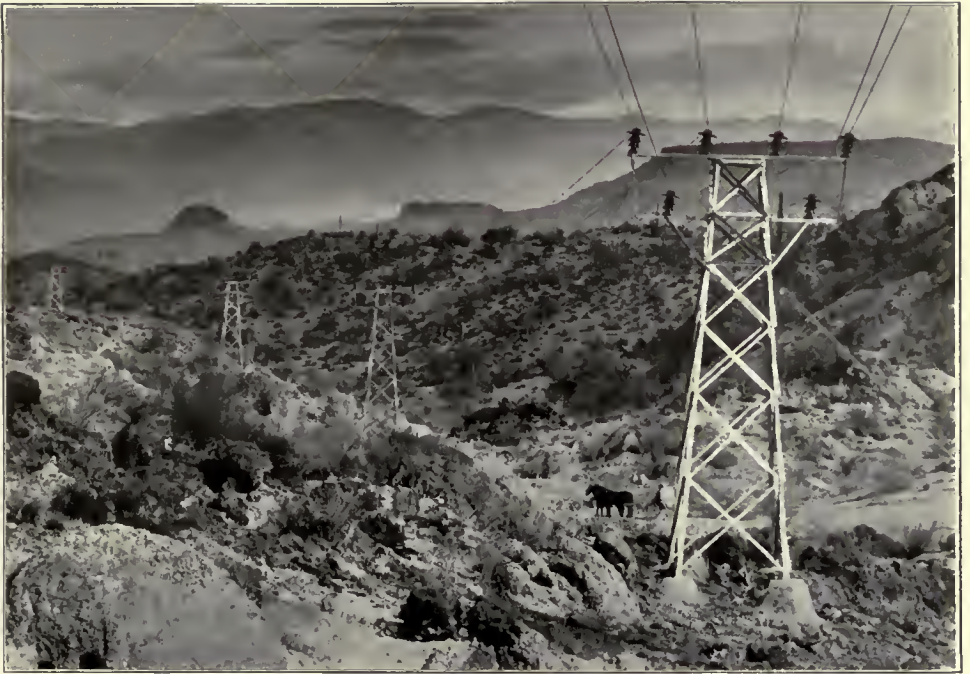
POWER LINE THROUGH SUPERSTITION MOUNTAINS, ARIZONA
