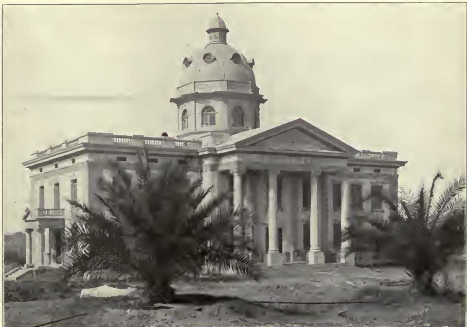
YUMA COUNTY COURTHOUSE, YUMA
