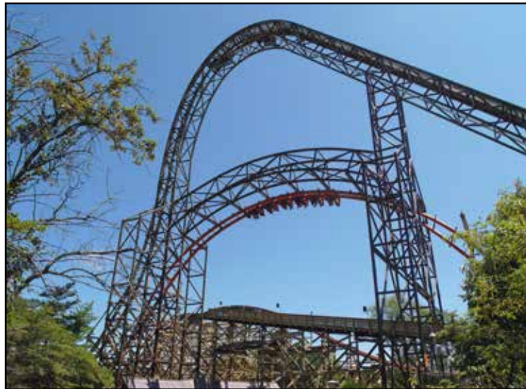
Seen above is the sleek, towering structure that provides Goliath with a steep 165-foot lift; the world record 85-degree, 180-foot drop; and the upside down span of the zero-G stall. Goliath features two inversions and three dramatic overbanked turns. At right, riders cheer for the exhilarating airtime moments incorporated into the 3,100 feet of track. The ride was built from the ground up utilizing Topper Track. AT/TIM BALDWIN
