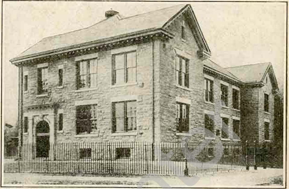
The modern consolidated school, or the type shown above, has come to stay. One such building takes the place of a dozen or more of the old type and makes possible thorough and capable instructing of the rural young Americans.
