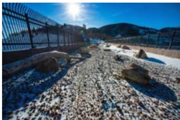
Source: Rick Egan | The Salt Lake Tribune. The first overpass for wildlife at the summit of Parleys Canyon crosses I-80 near Exit 140. Wednesday, Dec. 12, 2018.
