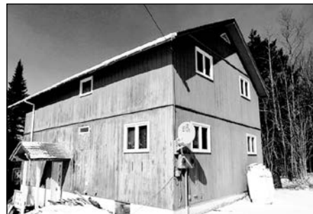
LOWELL A remodel for you to finish – 4 BR/1.5 BA, 6.6A, stone fireplace, gas heat, full unfinished basement. $59,000. Bruno. #4622958
