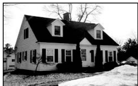
DERBY LINE. 1930's cape with hardwood floors, fireplace, 2 car garage, 2 baths, and eat-in kitchen. $139,000.
