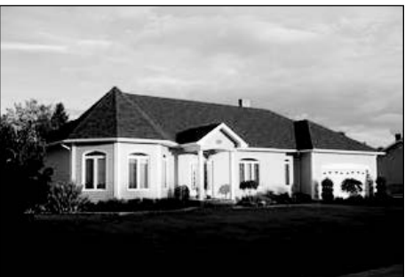
JCR 4759 ~ Newport: Quiet elegance! Immaculate contemporary with high-end materials & superb craftsmanship. Radiant heat, A/C, heated & insulated garage & landscaping like the professionals. 90 minutes to Montreal & 20 minutes to Jay Peak Resort. MLS 4483728. $263,900.
