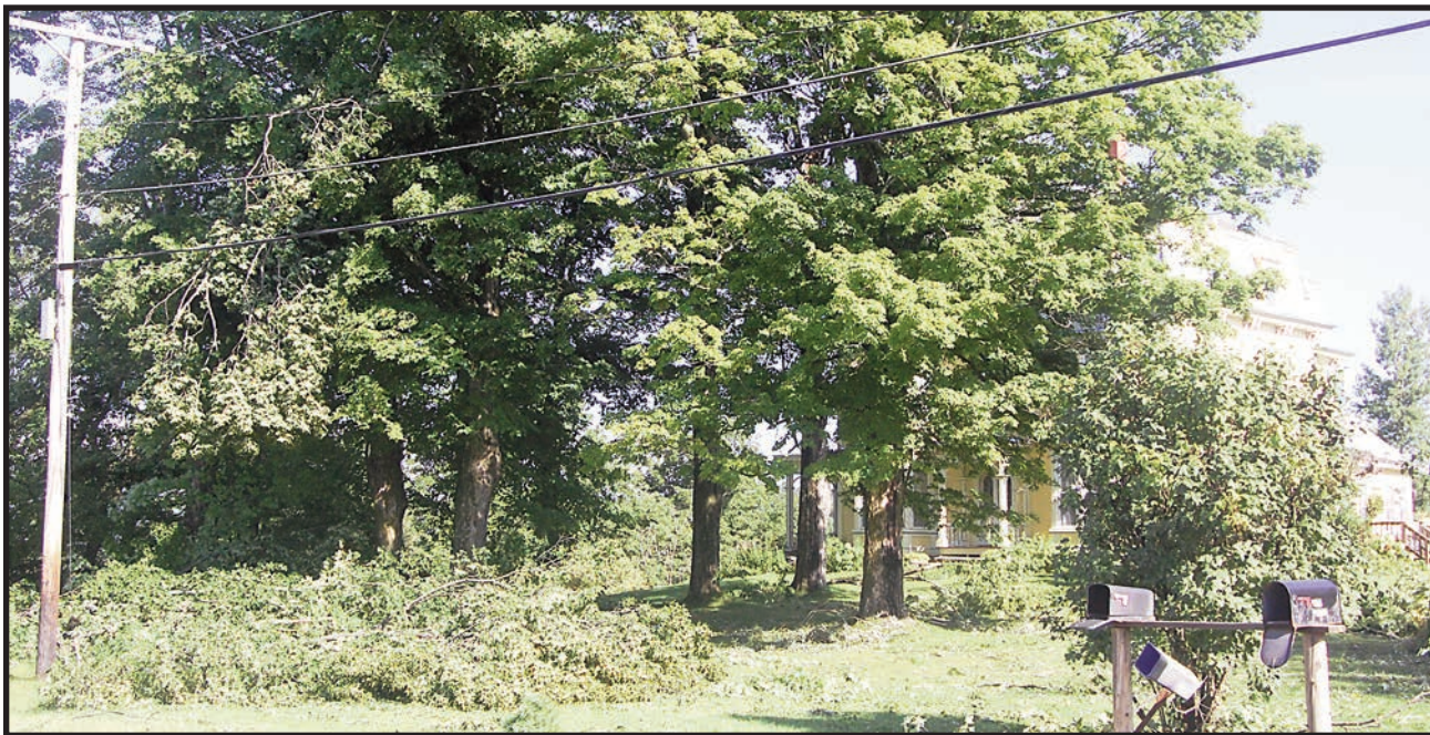
The two big, three-storied mansard roofed homes on Route 14 in Irasburg were hit hard by Monday's storm. Trees were blown down in both yards, which are generally beautifully landscaped. Photo by Tena Starr
