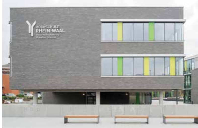
One of the new buildings opened in April 2014.
