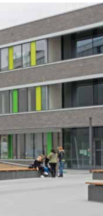
The new buildings of the Kamp-Lintfort campus designed by the general planner pbr AG.
