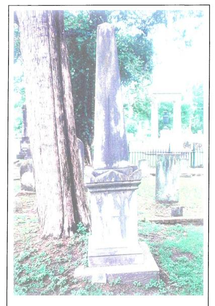
Figure 15. Example of leaning obelisk (Lot7). This stone will need to be disassembled, a foundation established, and the stone erected again.
