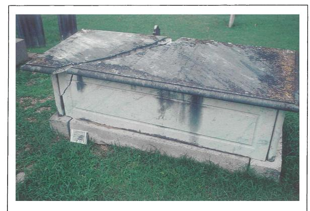
Figure 18. Box tomb with foundation problems causing damage to the side and top ledger (Lot 20). This is one of the more complex repairs.
