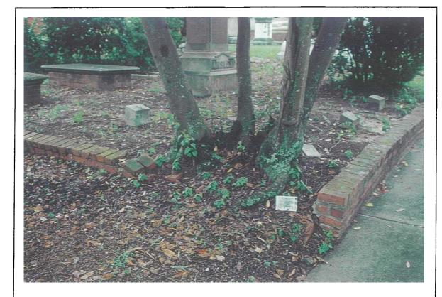
Figure 8. Example of "weedy" tree species growing from suckers off earlier cut stumps (Lots 13/14). Unattended these trees have caused extensive damage in this brick wall. These trees should be immediately removed, the wall taken apart and rebuilt to preservation specifications.
