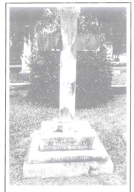
Figure 13. Example of a large cross (Lot 9) which requires resetting using a stainless steel dowel. These large monuments are of special safety concern.
