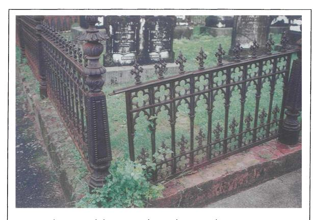
Figure 30. Iron fence segment which requires reattachment to the corner newel post (Lot 30). Vegetation growing along the base of the fence and on the brick wall should be removed.
