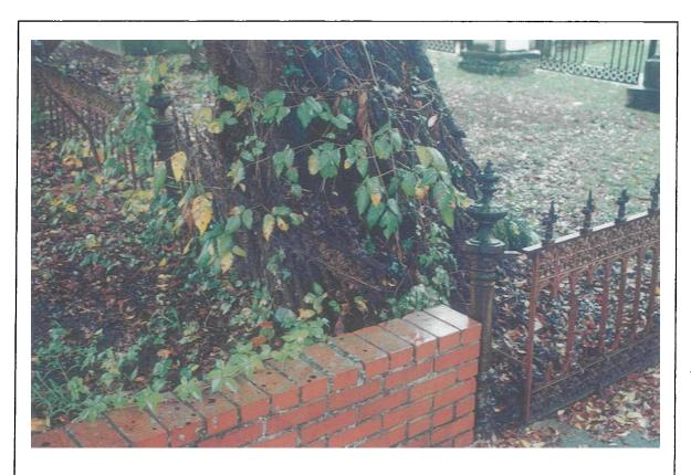
Figure 29. Example of tree which has been allowed to damage a fence segment (Lots 16/17). In this case the only choice is to remove the fence section and place it in storage. The aisle way segment should also be reattached to the corner newel post. This photograph also illustrates the large quantity of poison ivy which has been allowed to grow unchecked in the cemetery. This must be removed before any ironwork can begin.
