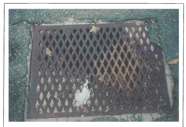
Figure 10. Example of a clogged drain. Other drains are completely clogged and some even have vegetation growing in them. These need immediate cleaning and repair.
