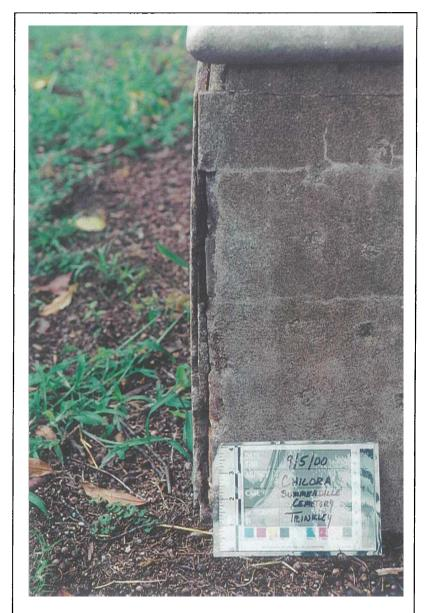
Figure 4. Example of stucco failure on a box tomb (Lot 23). This photograph shows at least two layers of a hard concrete stucco in failure with typical cracking and delamination.
