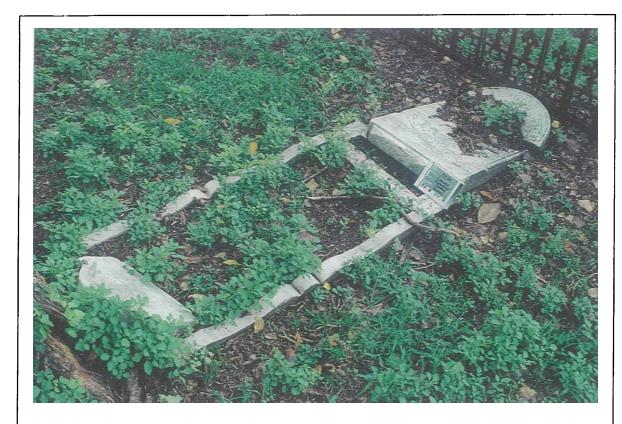
Figure 19. Collapsed headstone of a cradle grave (Lot 24). This illustrates why resetting intact loose monuments is so critical. Had this stone been reset before it fell, no costly repairs would have been necessary. Now, it will be necessary to drill and pin this stone, then reset it in the cradle tab — a more costly and time consuming operation.
