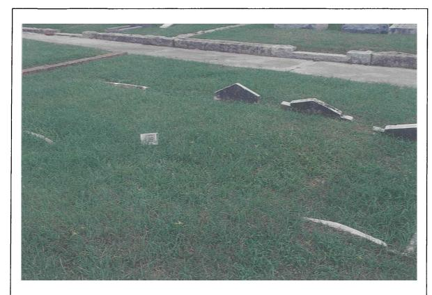
Figure 24. Example of simple cradle graves almost entirely lost below grade (Lot 65). Here it will take extensive, but careful, excavation to reveal the cradles before they can be raised to their proper level and set on better foundations.
