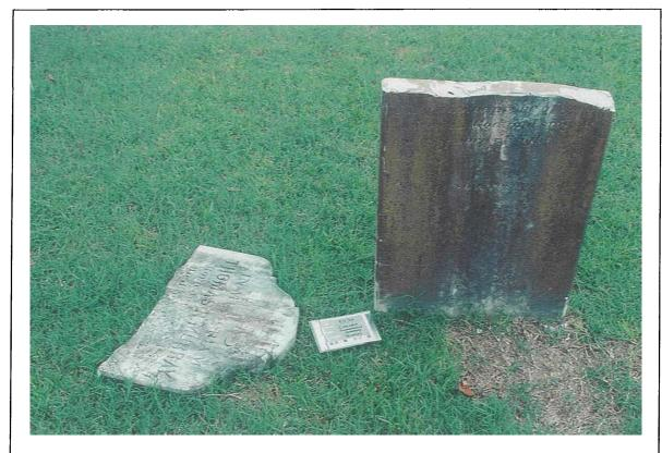
Figure 20. Example of simple headstone repair (Lot 56). This stone will require drilling and insertion of nylon pins for support.
