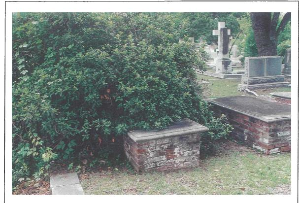
Figure 6. Example of unpruned plant taking over Lot 40. This azalea needs careful pruning for both its health and also to remove it from the box tomb. This dense vegetation will ultimately result in deterioration of the marble and the mortar joints.
