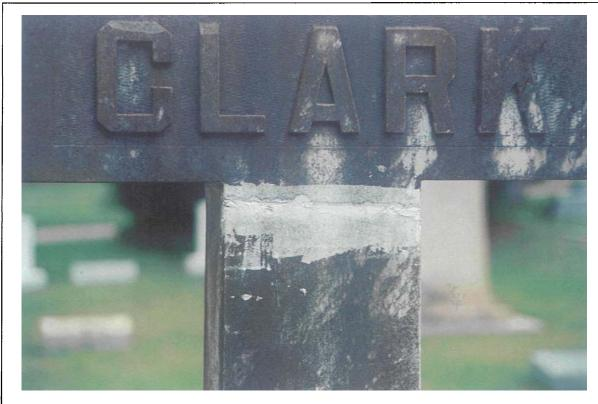
Figure 1. Example of unprofessional repair (Lot 191). Not only is there no documentation of the repair materials, but the application itself is sloppy and unprofessional. This is an example of the type of "repair" that the Trustees should eliminate from Summerville Cemetery.
