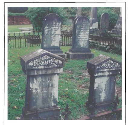
Figure 14. These four stones are all loose on their bases (Lot17) and require resetting using a wet, high lime mortar.
