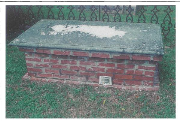
Figure 2. Rebuilt box tomb (Lot C). The use of modern brick and hard mortar, coupled with a lack of care in finishing the joints and cleaning the brick has resulted in an inappropriate "restoration" that detracts from the historic integrity of Summerville Cemetery. Such work should not be allowed.
