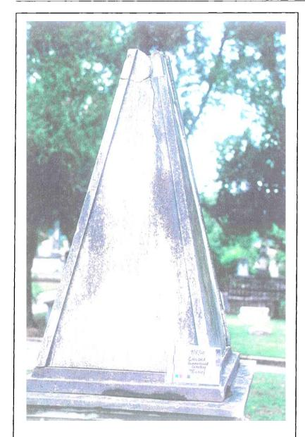
Figure 22. Example of obelisk which requires closure at the tip.
