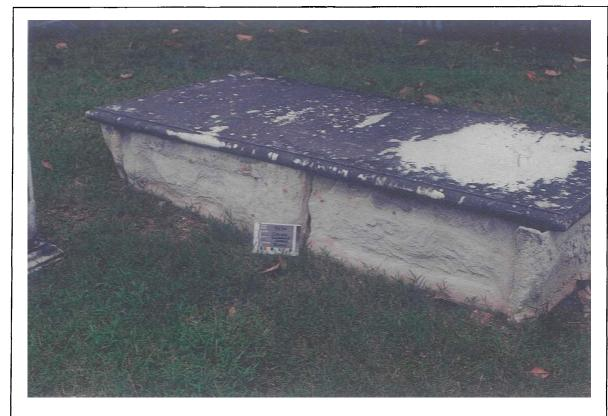
Figure 28. Box tomb with severely spalling sandstone sides (Lot G). In cases of such severe exfoliation the only approach is to use composite repair with is intended to provide a sacrificial coat.
