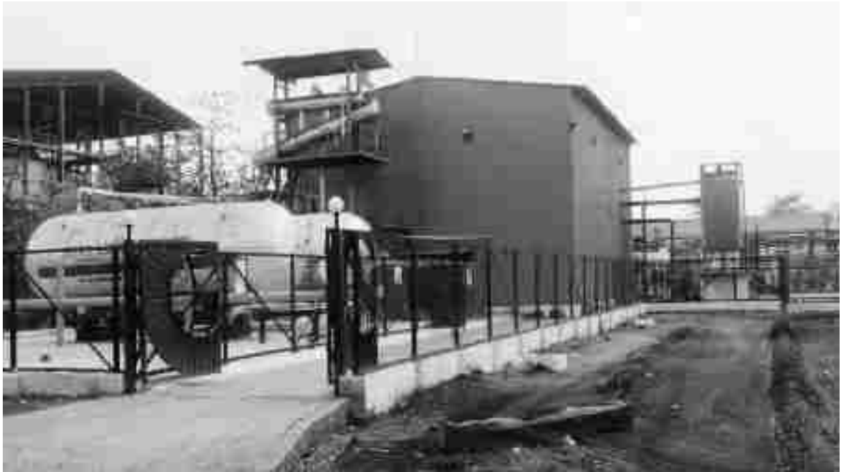
Pic-14 CO 2 Plant
