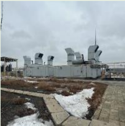
1. Pathway leading to main generating station
