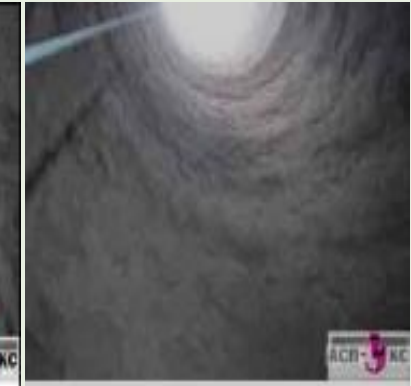
8. Accumulation and formation of layer of ash deposits inside chimney 3
