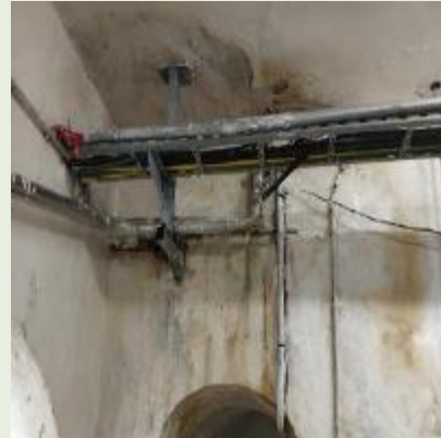
9. Fire extinguishing system in main transformer unit : seepage of water observed
