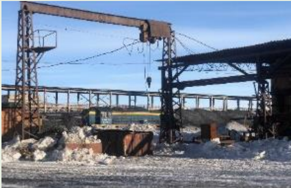
1. Open coal storage yard – coal is exposed to snow and ambient conditions
