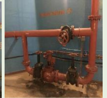
3. Fire fighting system: well maintained with no observed leakages or cracks in the structures.
