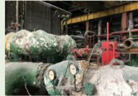
3. Insulation damage
