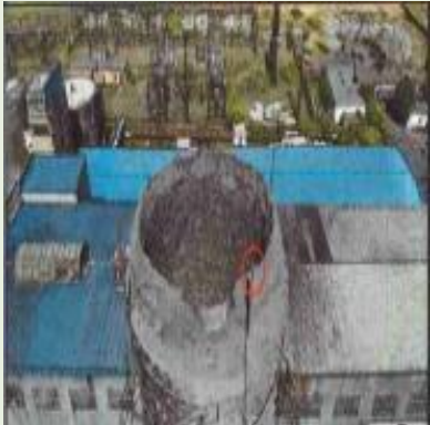
1. Poor condition of chimneys 2
