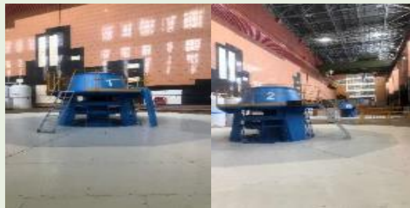
2. Turbine halls were well maintained
