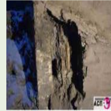
6. Destruction to the protective concrete layer 3
