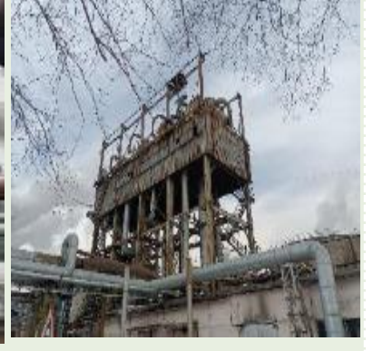
3. Rusting of piping, equipment
