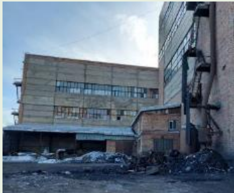
9. Outside of BTG house : wasted coal and metal debris dumped
