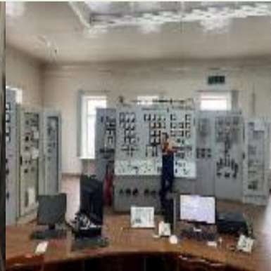
7. Analog metering/ knob type manual operation desk 2
