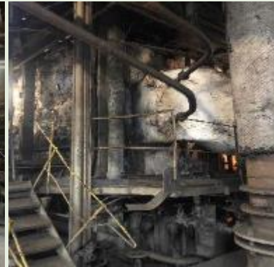
2. Cracks on floors and structures along with coal dust deposit.
