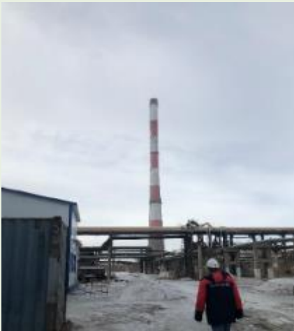
1. Power plant chimney
