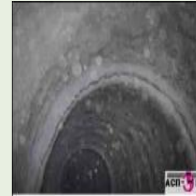
8. Accumulation and formation of layer of ash deposits inside chimney 3
