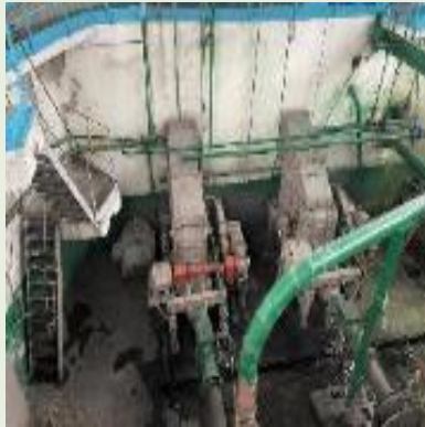
4. Water spillage & algae grown in pumping area 2
