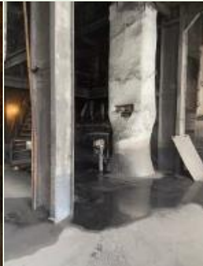
1. Water and coal dust leakage
