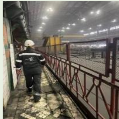
2. Cracks on floors and pathways
