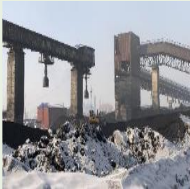
1. No dust and fire suppression system
