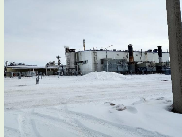
3. Back-up turbine generators
