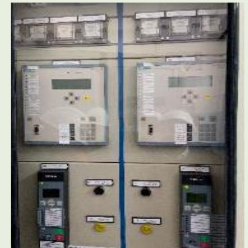
4. New numerical relays
