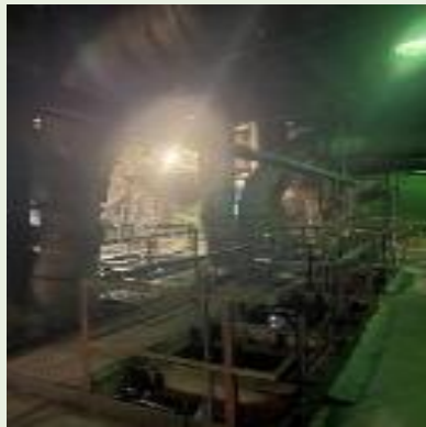
4. Coal dust accumulation on equipment
