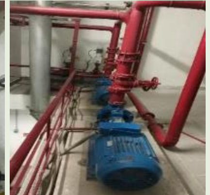
9. Fire extinguishing system in main transformer unit : seepage of water observed
