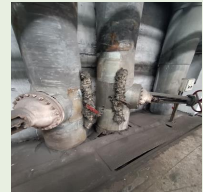
6. Damaged insulation
