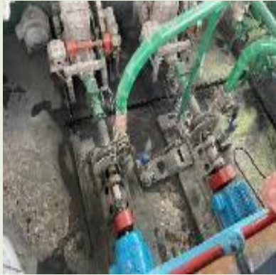
4. Water spillage & algae grown in pumping area 2
