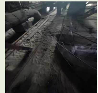
3. Fly ash covered the boiler floor
