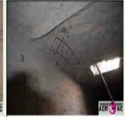
6. Destruction to the protective concrete layer 3
