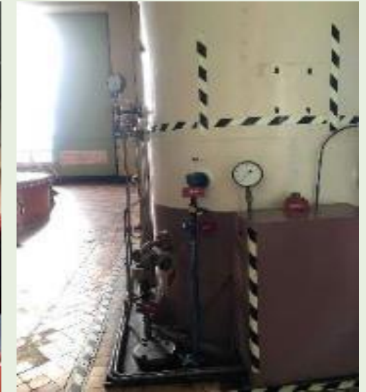
3. Missing pathway markings and floor tiles damaged
