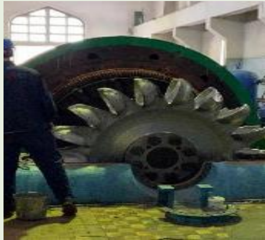
2. Hydro turbine under maintenance
