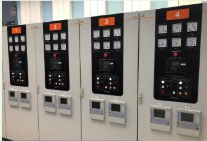
2. Numerical relays for generation protection
