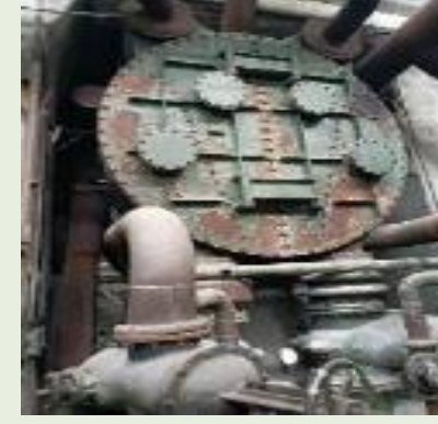
3. Rusting of piping, equipment
