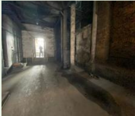
1. Water and coal dust leakage
