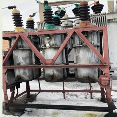
2. Oil leakage
