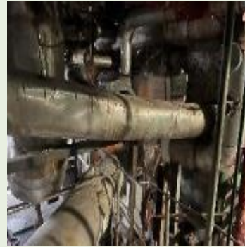
2. Extensive damage to the insulation/ missing aluminum cladding 2
