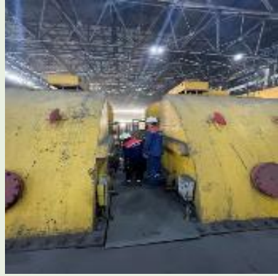
1. High amount of coal dust deposit and debris accumulation seen
