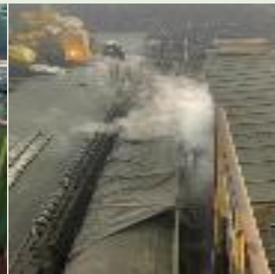
3. Steam and water leakages
