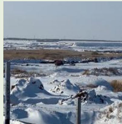
5. Ash dump 2: under construction
