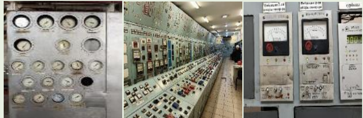
7. No DCS and analog control systems used in the control room
