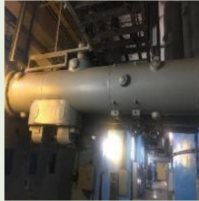
2. Main busbar: MARKS and dents observed
