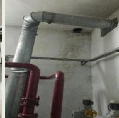
9. Fire extinguishing system in main transformer unit : seepage of water observed
