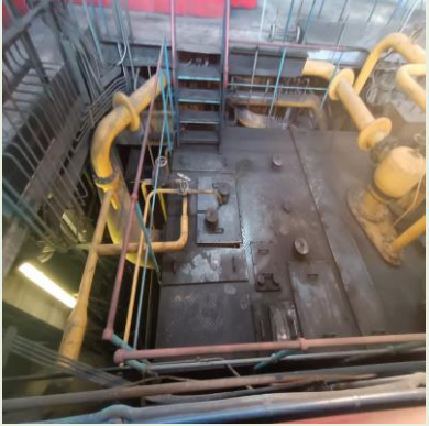
1. Coal dust accumulation over lube oil tank
