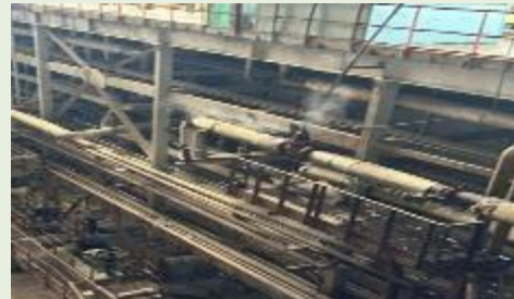
2. Steam leakage
