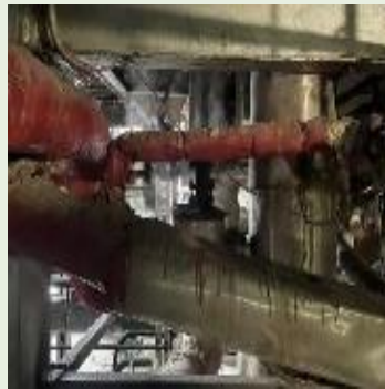
2. Extensive damage to the insulation/ missing aluminum cladding 2
