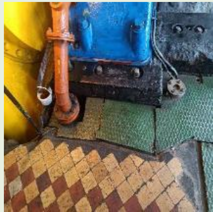
1. Water and oil leakages
