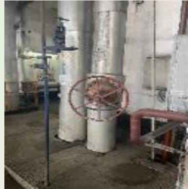
2. Rusting of pipes and equipment
