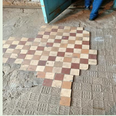
6. Flooring damaged
