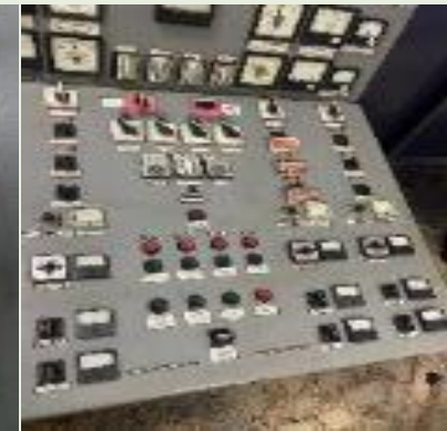
5. Manual / semiautomatic control center.
