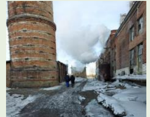
11. Chimney area: Continuous blow down vessel of boiler not insulated
