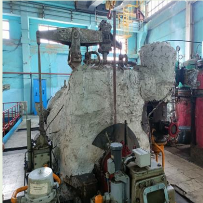
5. Damaged insulation in boiler-turbine
