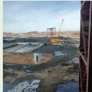
7. Open coal storage yard
