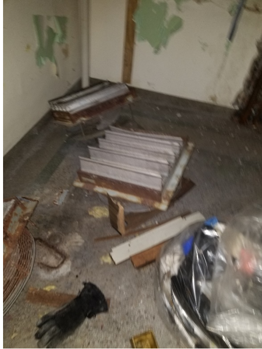
Wall Mounted Fans
