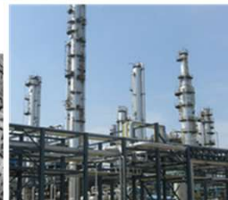
Air Liquido Engineering & Construction, Rectisol™ - Syn gas cleaning
