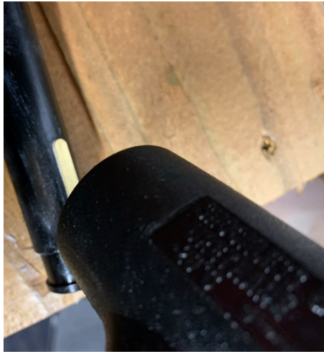
31. Refit brass keys and use a hammer to hit into place.
