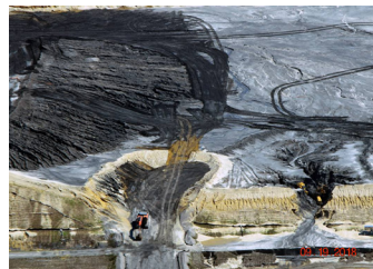
Coal ash pond spill near Wilmington, North Carolina 53
