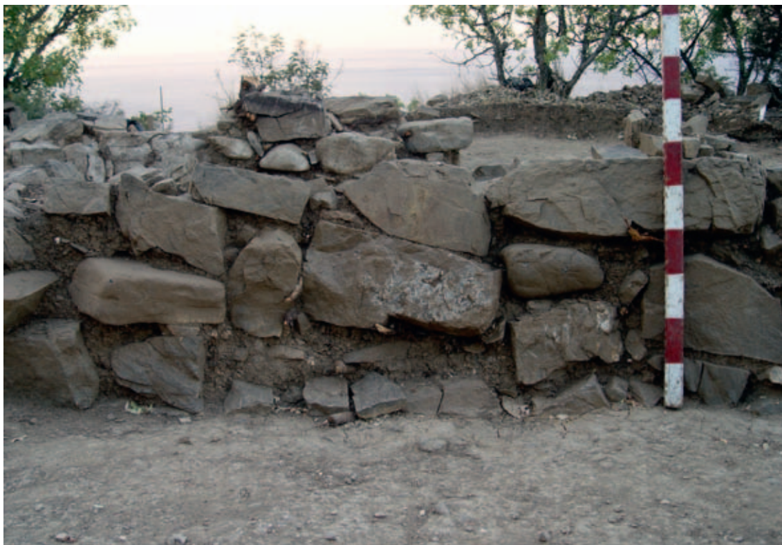
Рис. 1.21. Северный вход в храм. Закладка проёма в третьем строительном периоде. Вид с юго-востока. Fig. 1.21. Northern entrance to the church, closing of the doorway between northern and southern parts of the church in the third building period, view from southeast.
