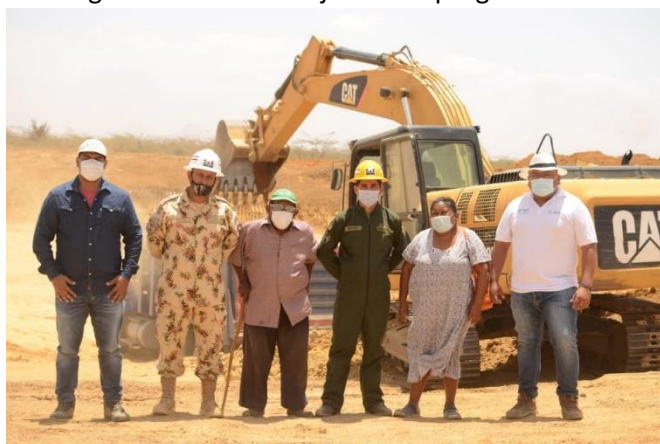
PAR and Enel in coordination with the National Army's Engineering Command constructed community dams in Guajira
