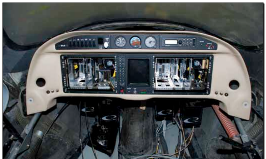
The beautiful Evolution instrument panel doesn't look as nice stripped of its major components, but the weight savings makes handling much easier and prevents possible damage to the expensive Garmin boxes that will go in later. Cannon plugs that connect to pre-made wiring harnesses make panel installation easier than you might think.
