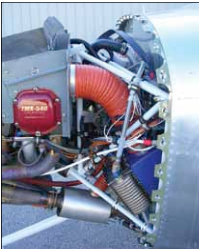
Even with simple installation, the firewall-forward area of your plane can become quite crowded, which makes routing of wires even more important for safety, reliability and future maintenance.
