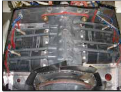
Routing of spark plug harnesses secured through baffle materials.
