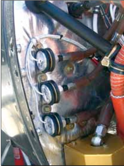
Alternative mounting for probes and sensors on this composite firewall.
