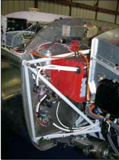
Firewall forward view showing the battery box and relays as well as a ground strap on the engine mount.
