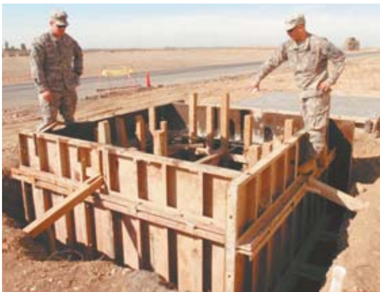
Capt. James Pascoe, right, commander, Headquarters and Headquarters Troop, 2nd Squadron, 6th Cavalry Regiment, Task Force Wings, explains the concept of a black water and fresh water pit at Forward Operating Base Warrior, near Kirkuk, Iraq, Nov. 15. The pit is part of an ongoing life support construction project totaling between $2.5 to $3 million for the squadron's troopers.
