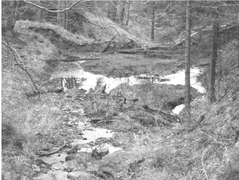
Figure 5: Material accumulated upstream of one of the dams in Cerny Potok stream.
