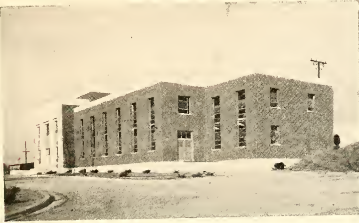
Filter Plant, New Water System
