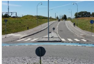
Road Safety & Accessibility
