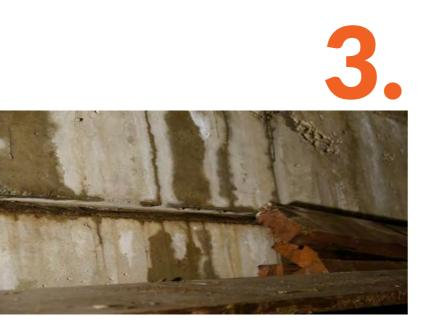
If a visual inspection of your crawl space shows water on the walls or floor, then moisture condensing on a cold surface might be the issue. Moisture from inside your home will condense on the cold foundation walls if crawl space insulation is inadequate. In summer, cold water pipes that are not insulated will condense water and will drip onto the floor.
