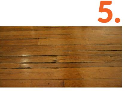
Sagging or warping floors are serious signs of crawl space problems, and it's likely they've persisted for years. What's happening is that your floor joists are deteriorating or moisture is warping the subfloor. There are many causes of floor joist damage including rotting wood from excess moisture and damage from termites and carpenter ants that are attracted to the moisture.
