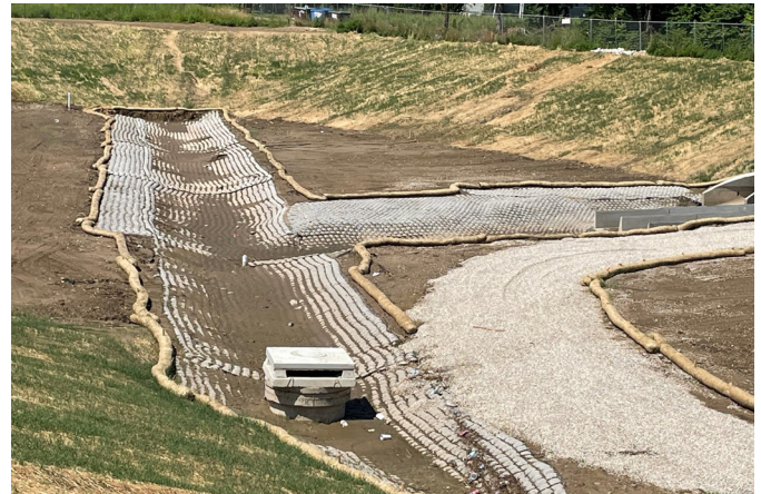
Flexamat installed in the water flow lines to prevent erosion. The site received a lot of rain after installation, so straw wattles are used to keep the mud off the Flexamat.
