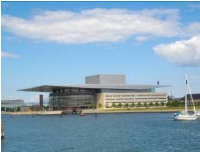
Copenaghen Opera House
