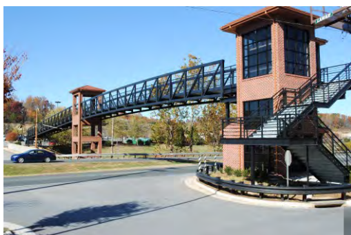
Pedestrian bridge across Ward Road provides safe access
