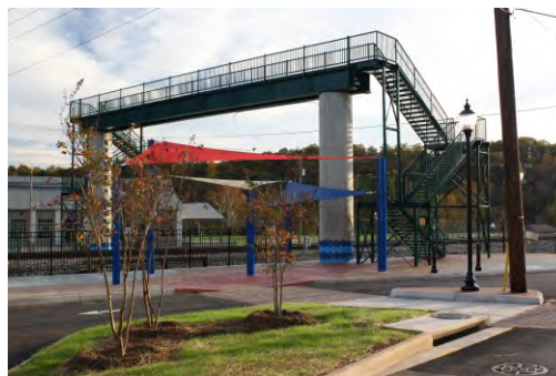
Altavista pedestrian bridge highlights historic and cultural connection to the Staunton River
