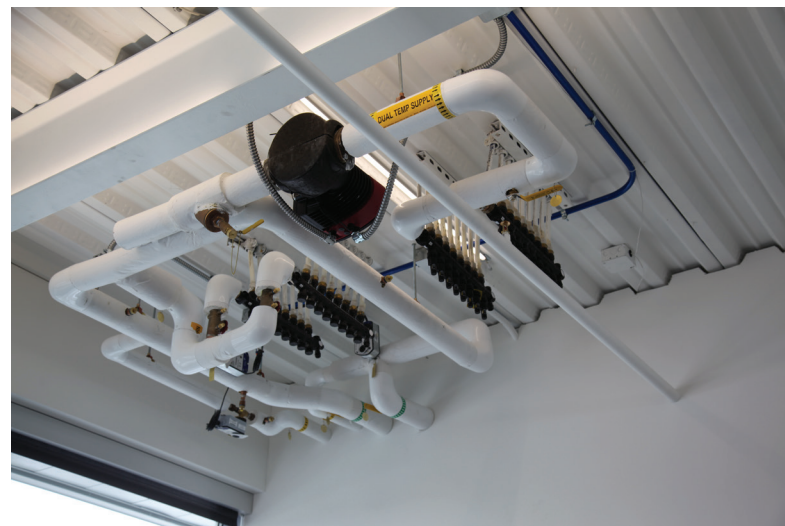
Detail of the radiant heating/cooling tubing and manifolds driven by a VSD pump.
