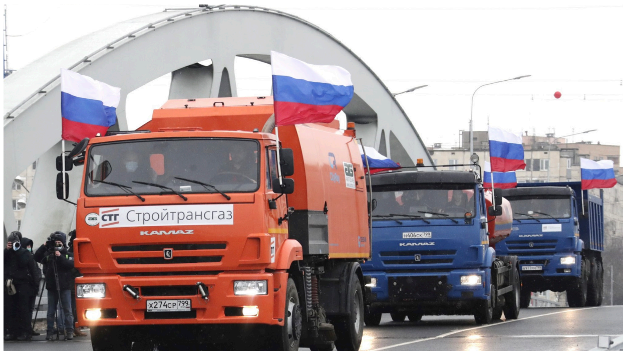
Building equipment at a newly completed interchange along Russia's M10 highway in January of 2021. (en.kremlin.ru)
