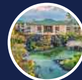
GRAND HYATT KAUA'I RESORT & SPA: 604 ROOMS
