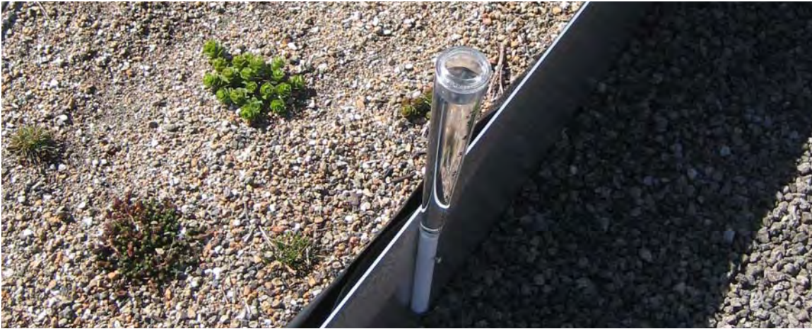
Figure 4-20: Rain gauge at PS118 in Queens.
