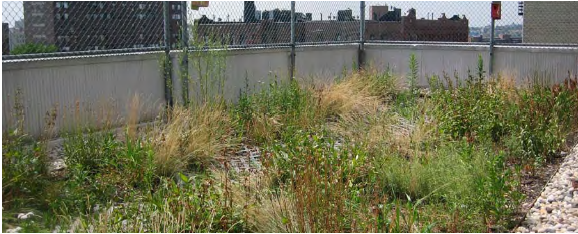
Figure 4-18: Fence installed on St. Simon Stock School in the Bronx to allow student access to the green roof.
