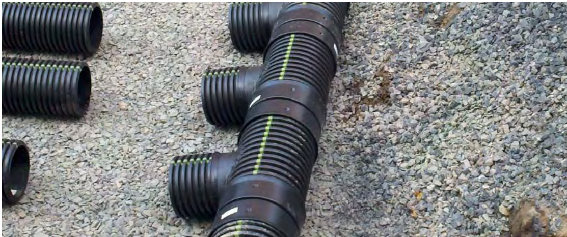
Figure 3-11: Manifolds can be used in subsurface systems to evenly distribute flow through the system.
