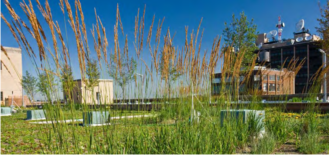
Figure 1-4: The largest green roof in New York City, approximately 2.5 acres, is on the Morgan Mail Processing Facility in Manhattan. (Source: United States Postal Service. All rights reserved. Used with permission.)
