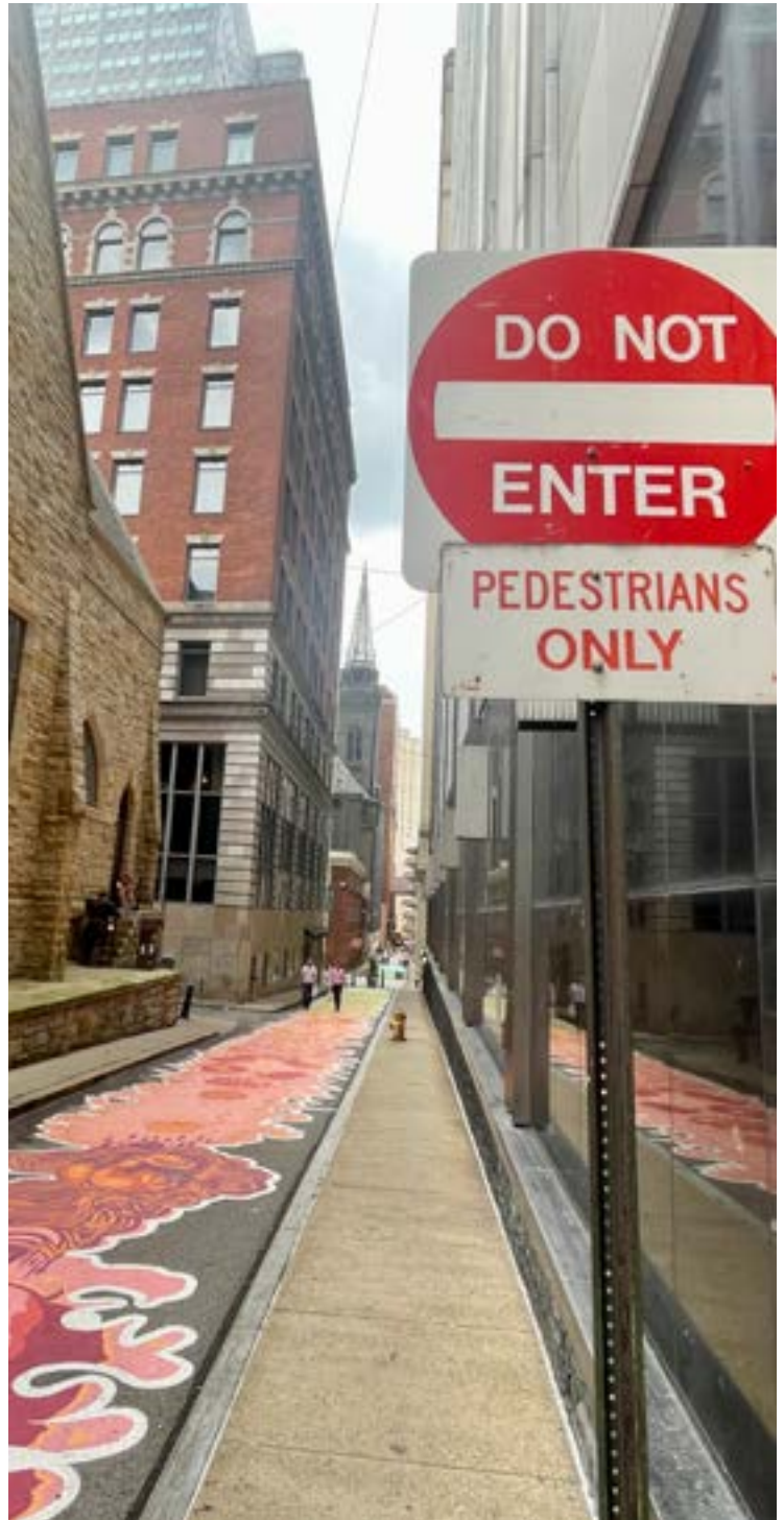
Alley Renovations on Cherry Way.
