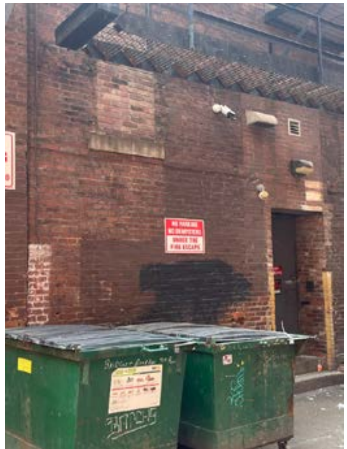
Dumpsters under the fire escape, directly under the "no dumpsters under the fire escape" sign
