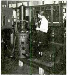
MAIN COVER FEATURE The new G.E. 100-kw. pliotron is shown here with its exhausting apparatus, and replaceable filament.
