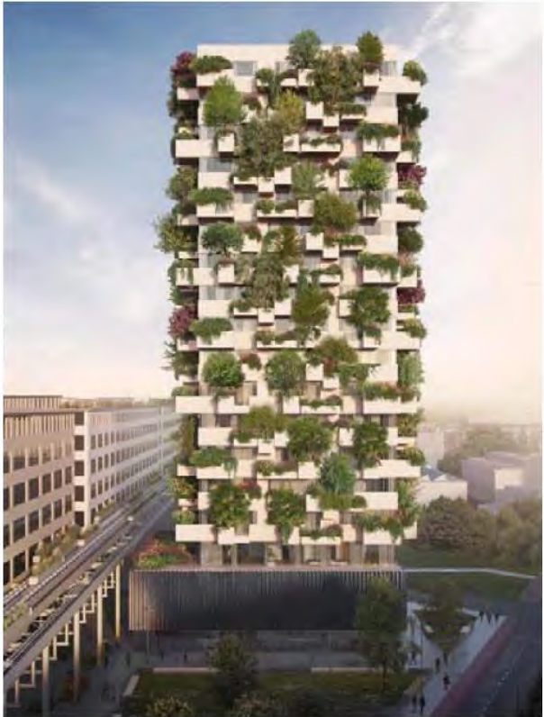
The Trudo Vertical Forest is the first to be adopted by a social housing project
