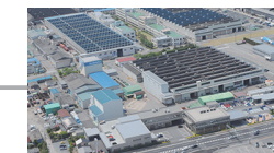
Utsunomiya South Plant/ 2nd South Plant
