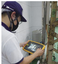
Air leak investigation
