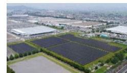
Japan’s largest-scale solar power system (Gunma Oizumi Plant)
