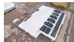
Installed at Subaru Accessory Center and others
