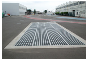
Flood prevention measure (drainage grid) (Utsunomiya Plant)
