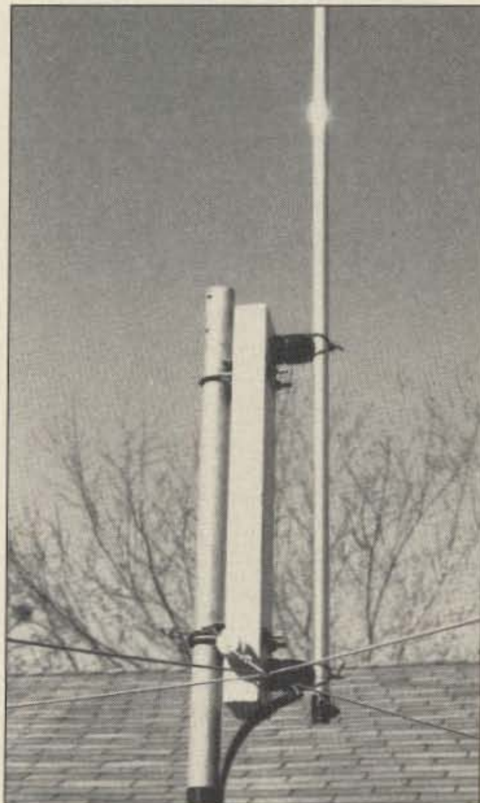
Connections should be soldered and protected from the weather with tape or silastic compound.
