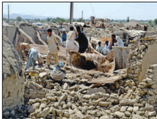
Destruction by earthquakes
