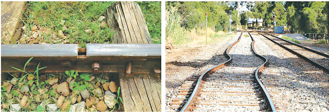
Expansion gap in railway track
