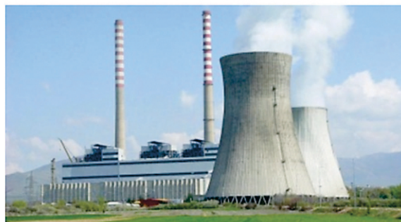
Figure 9.4: Thermal power plant
