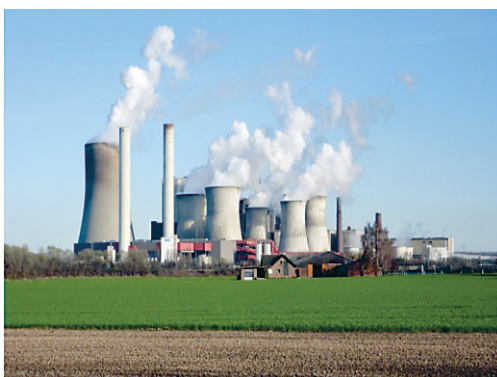
Smoke emitted from thermal power station
