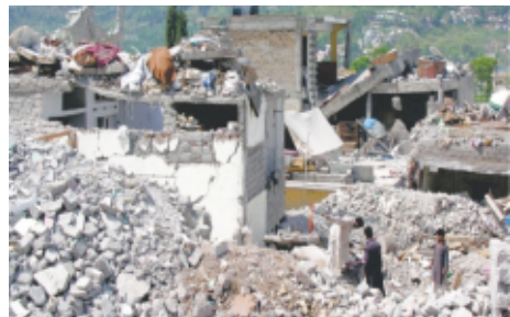
A view of earthquake destruction in Balakot
