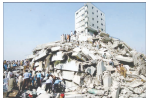
An view of destruction caused by an earthquake in Islamabad
