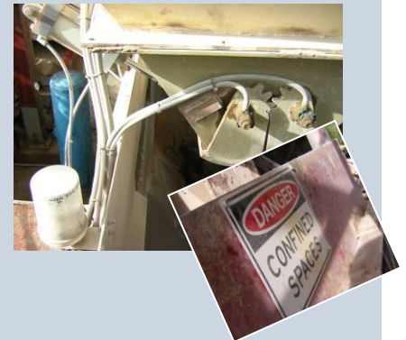
Load chutes with confined space entry
