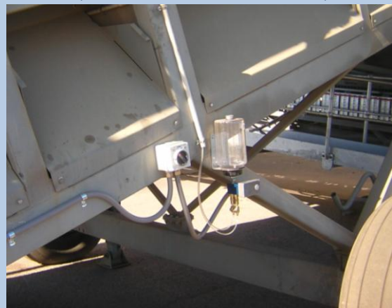
240V 4L Electric oil lubricator with 6 outlets installed
