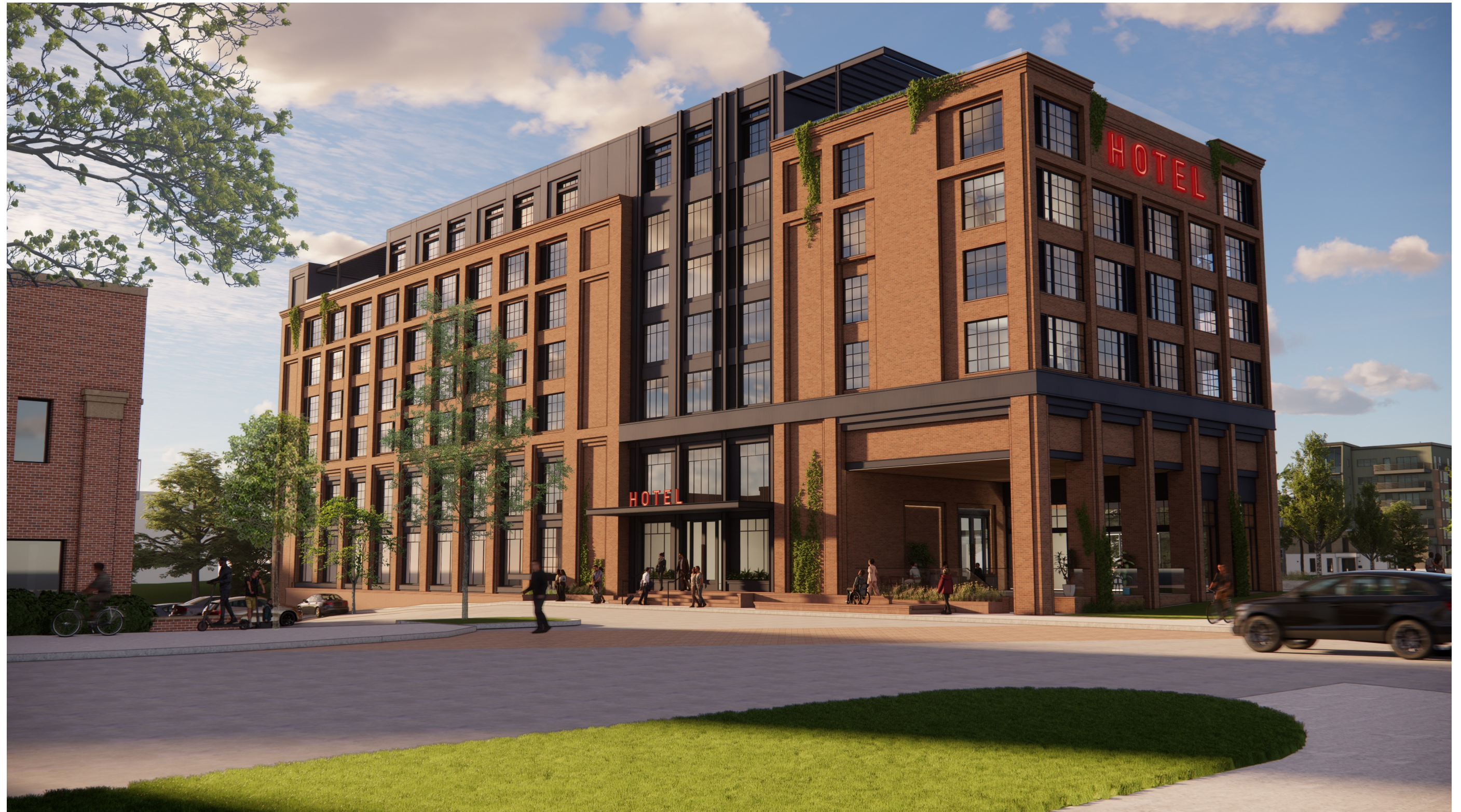
South Façade – Image looking northeast at the hotel main entry
