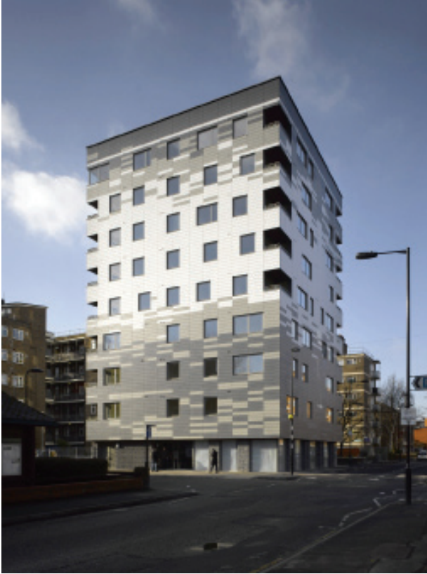
FIGURE 3. Murray Grove housing – The UK’s first urban high rise housing project to be constructed entirely from pre-fabricated solid timber. Image courtesy Waugh Thistleton, photo: Will Pryce.
