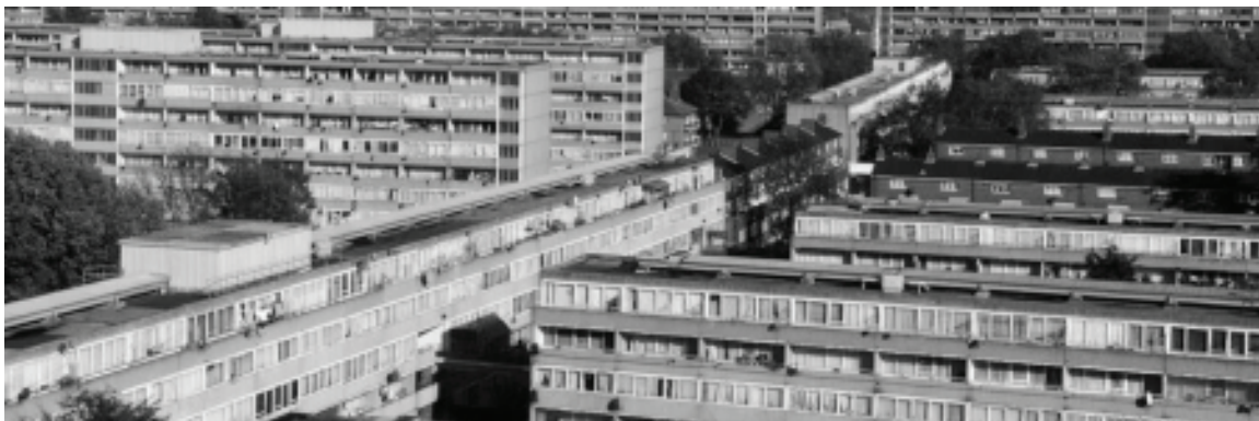
FIGURE 9. Type D. Elongated terrace housing - Gayhurst House, Aylesbury Estate SE17 2BL
