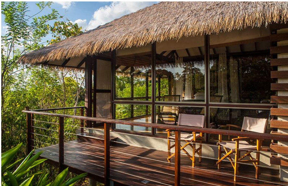
Ulagall Resort's features ecologically-built villas
